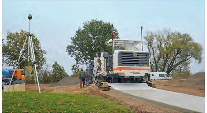
The AutoPilot steered the SP 25i from Wirtgen in the construction of the 3m wide dyke path by Böhling Bauunternehmung GmbH. The height was controlled by a laser transmitter with the appropriate receiver on the paver.
