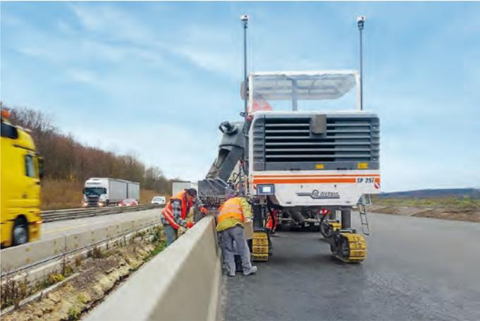
No stringline obstructed the construction of this concrete protection wall. The VSB infra construction team enjoyed the freedom of movement just as much as the concrete mixer drivers – they can manoeuvre in front of the paver much better without a stringline.
